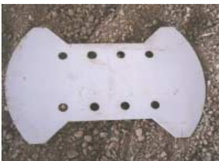
Fig. 1: This steel plate was located at the top of the columns in the new Pearson airport terminal and provided a location to connect to the roof trusses
