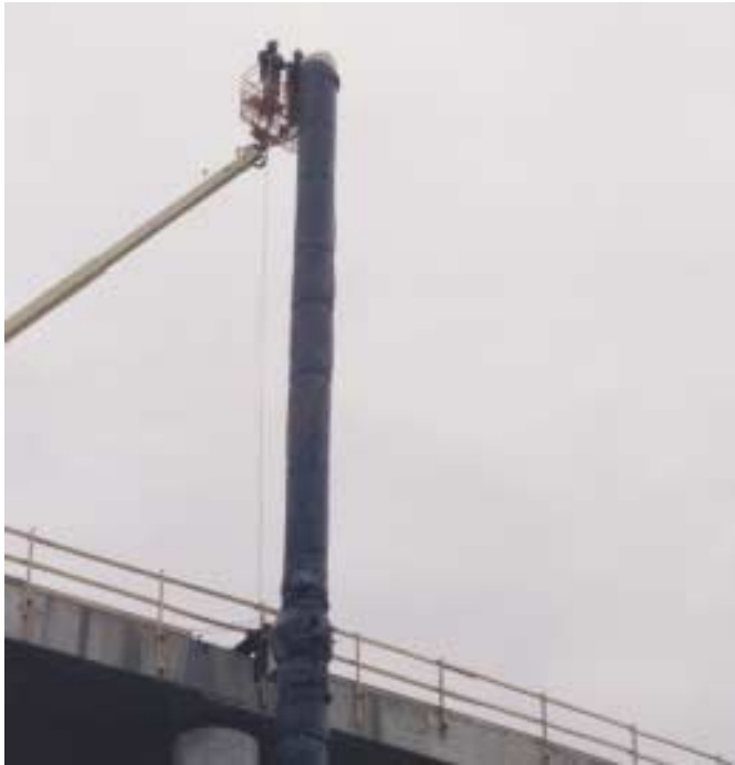
Fig. 2: Workers observe SCC placement in the test column to avoid overfilling
